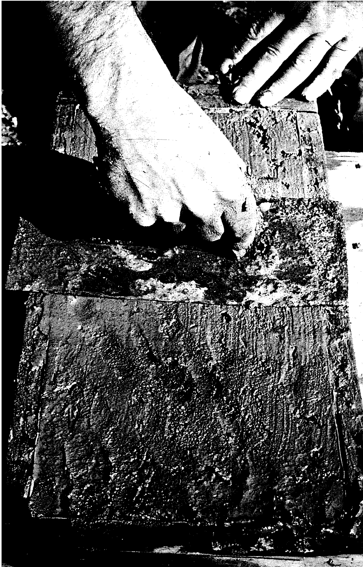
Using a trowel to strike the mud level with the top of the mold.
